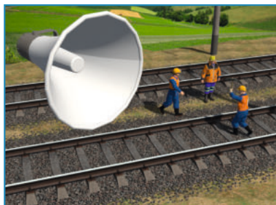
Warning of operating personnel about incoming trains
